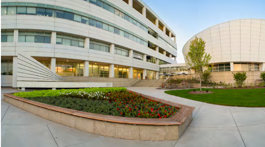
Building 401, one of six buildings included in Argonne's Smart Labs Program
