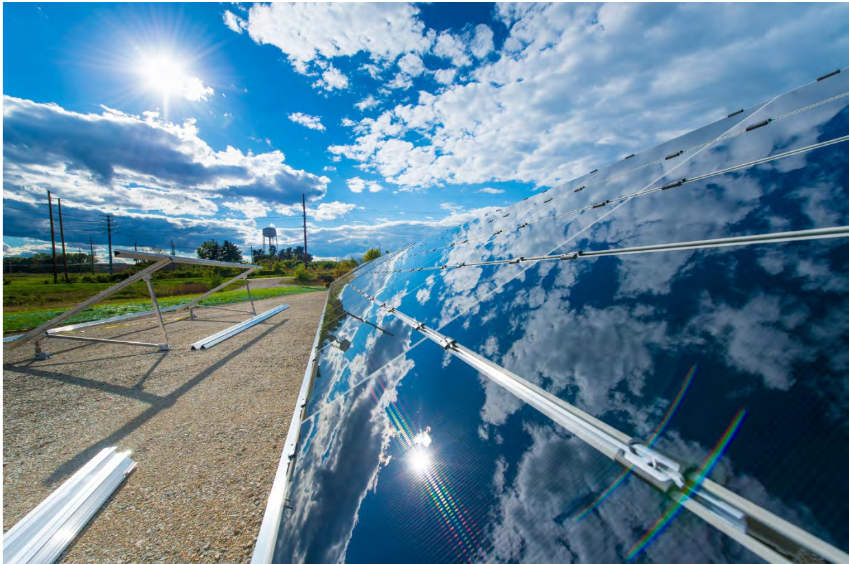
Figure 14: Building 372/373 Solar PV Array
