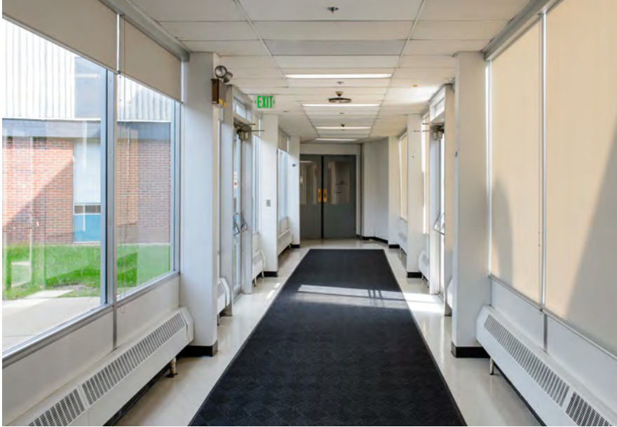
Adjustable fiberglass window shades installed in the corridor connecting Building 362 to the adjacent Building 360
