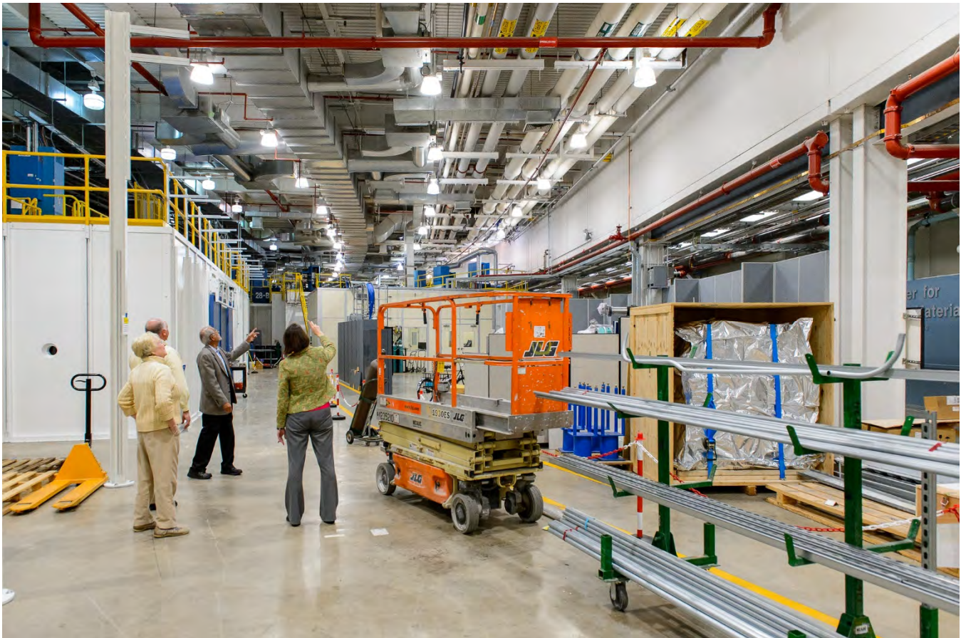
Figure 3: Project Team Reviewing Portion of Completed APS Experiment Hall Lighting Improvements
